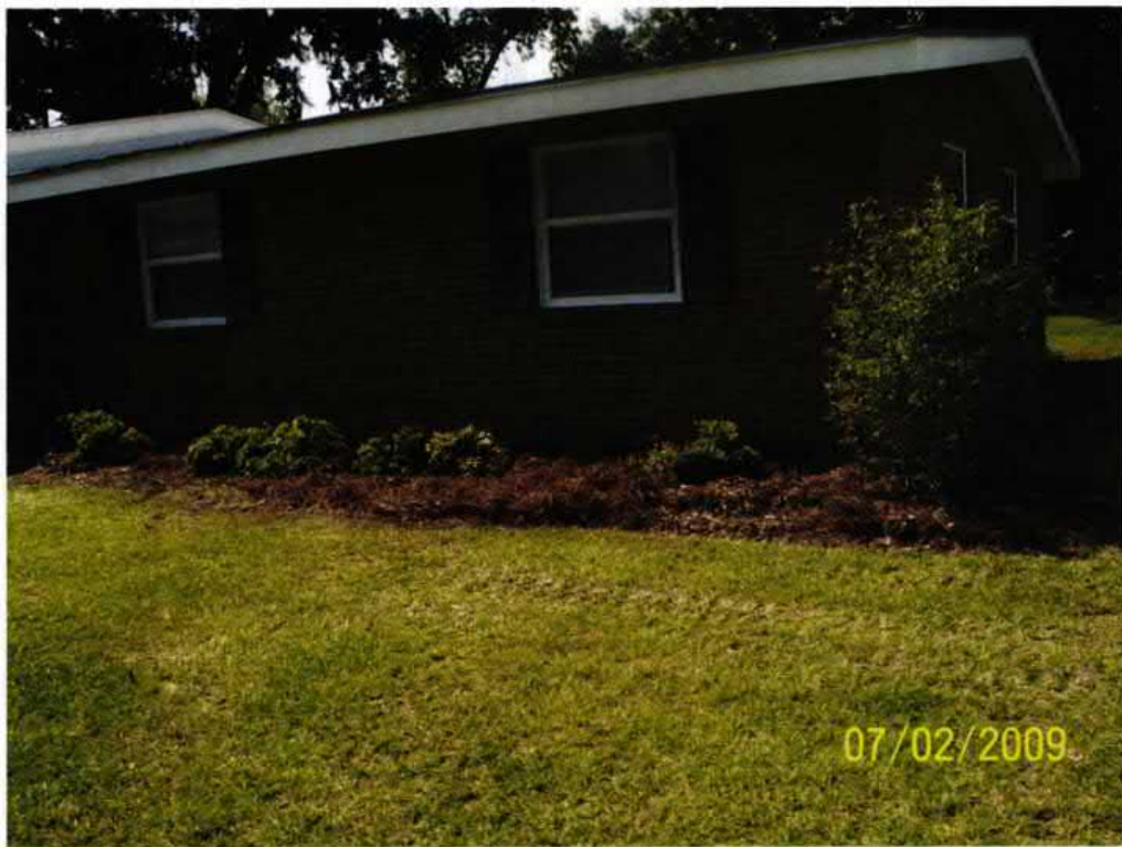
Picture 2: Site after completion of work.
